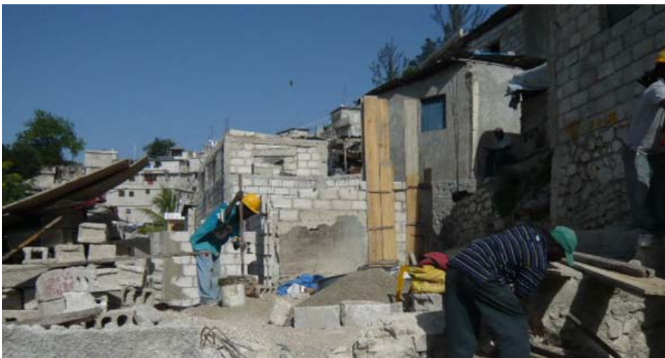
A home repair underway using the training and building guidelines taught by Build Change, June 22, 2011. Photo delegation.
